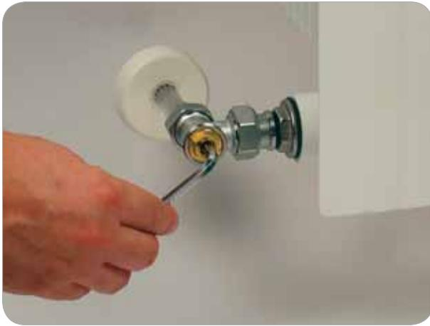
This operation, to make according to design characteristics of the system and of hydraulic characteristics of the product at issue, is crucial to guarantee the proper operation of the system. Removing the upper cap you can reach easily the adjustment rod that should be operated with the help of a specific hexagonal wrench (R73). Starting from the position of all closed the shutter is opened according to what the system design provides for.
