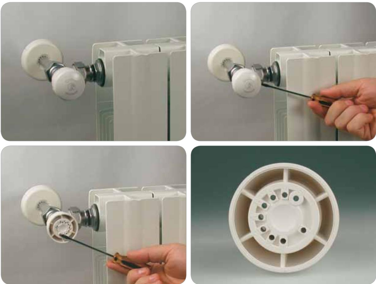
The adjustment can be made shifting the metal pin in the position that best suits one's needs, according to the specific diagrams reported in the [Hydraulic Versions and Characteristics](#).
